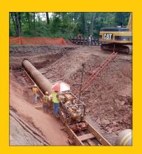
Horizontal directional drilling technology can be utilized for short or great distances. Installation lengths of up to 6,500 feet have been successfully installed with pipe diameters as large as 48 inches. Although directional drilling was originally used primarily through loose soils, more and more crossings are being undertaken through gravel, cobble, glacial till and hard rock.
